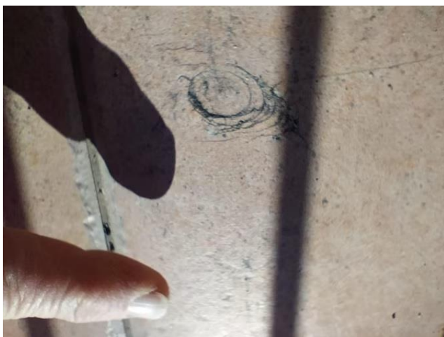
Figure 4 – The tile of the balcony damaged by the impact of the meteorite. (Credits: Prisma/Inaf).
