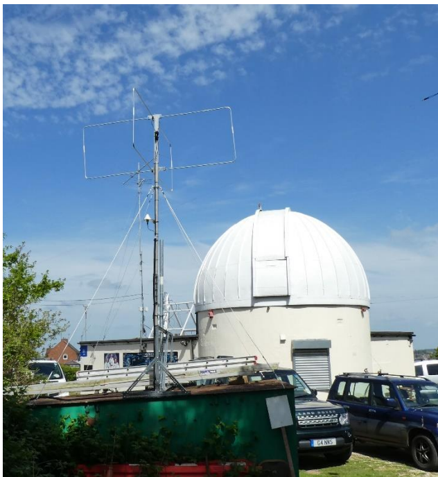
Figure 1 – The beacon installation at the Sherwood Observatory.
